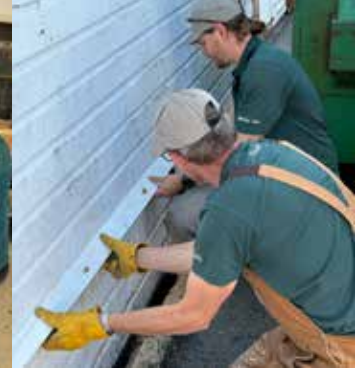
Parks Canada team repairs exterior wall of the Cannery. GOGCS photo.
