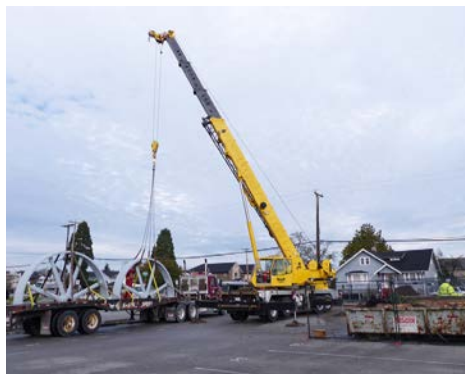
The Triumph Ice Machine is lifted by crane into its new location.
